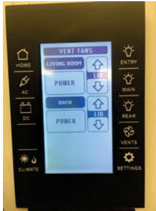
Figure VIII Remote Vent Fan Operating System
